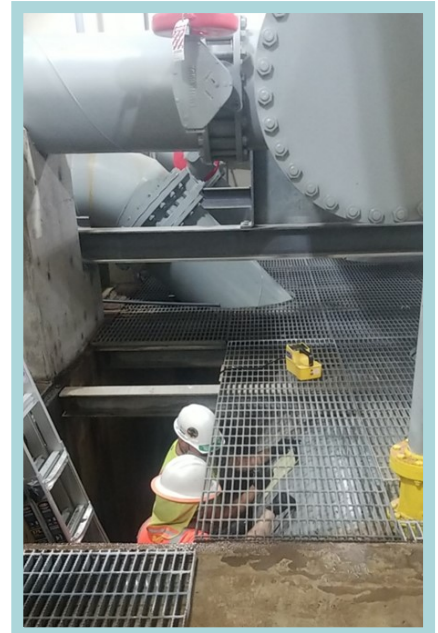
Technicians testing pipe thickness.
